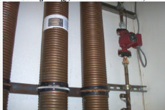
(b) Three speed Grundfos UP15-42F Circulator (Circulates cold & preheated water between 4 GFX-coils & 3 85-gallon gas water heaters @ 4.7, 5.8 or 6.5 gpm)
