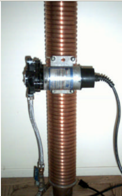
G3-60 GFX & Low Power Diaphragm Pump SHURflo Model 2088-594-500 Internal Check Valve, 80 Watts @ 2.4 GPM (115 VAC, 0.55 to 0.9 AMPS)
