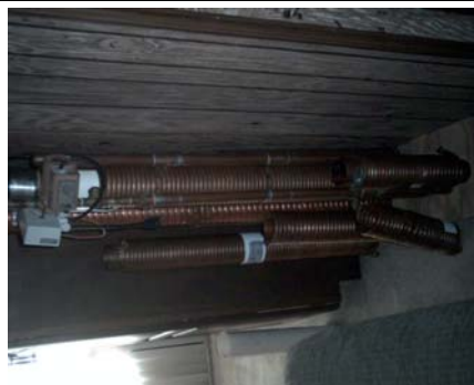
Fig. 4(b) Cut & intact Vaughn G3-12's. No continuous yellow stripe on 3" central DWV drainpipe.
