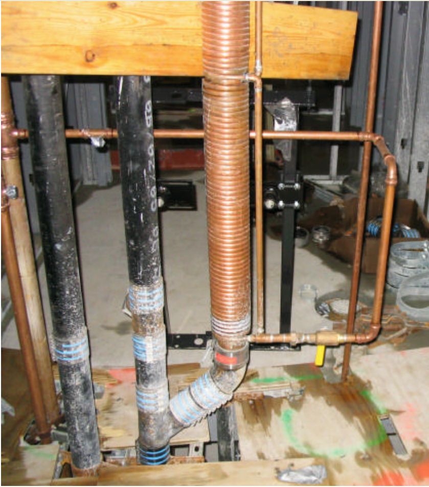
Fig. 1 GFX Model S3-60 in Dormitory Chase, Dartmouth College.
